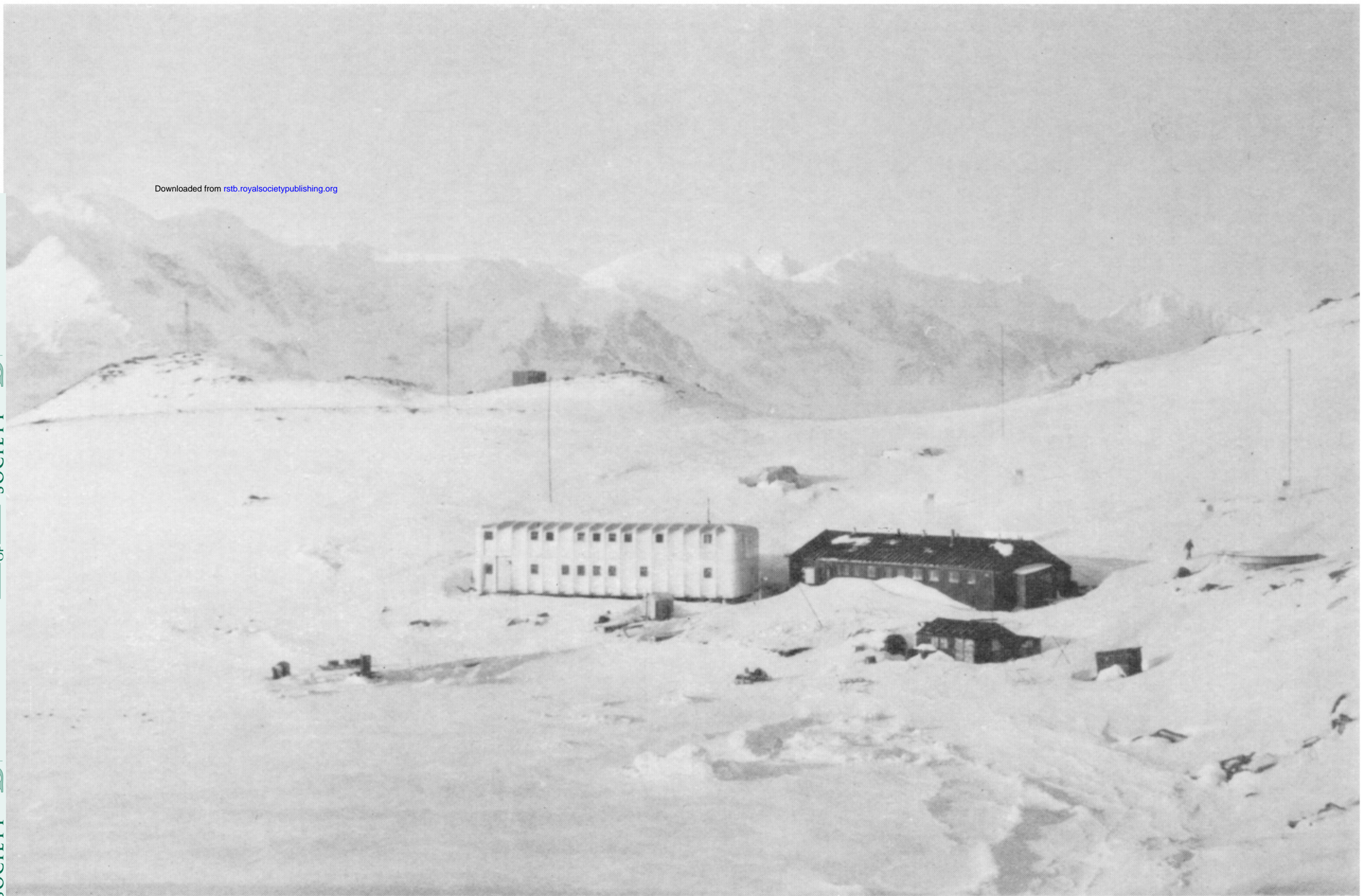
FIGURE 4. The new and old base huts on Signy Island. The prefabricated building on the left has a shell of resin and fibre-glass and provides laboratories on the ground floor and living quarters above.
